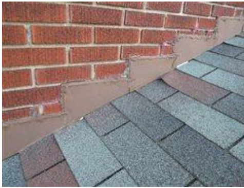
Photo 40 proper flashing installation
