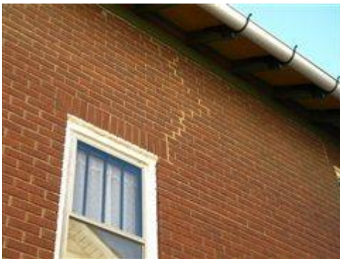
Photo 4 repaired crack
